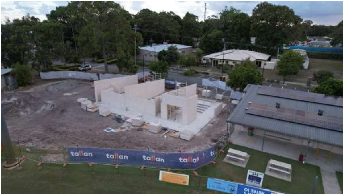
Overview of site
