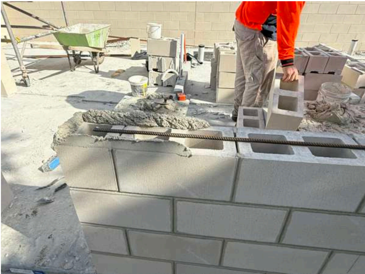
Horizontal steel reinforcement being installed during block wall construction
