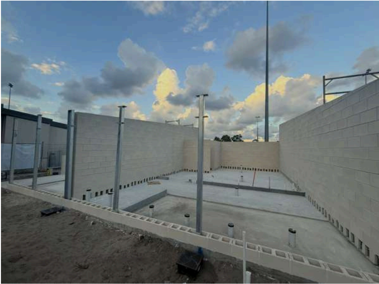
Blockwork nearing completion
