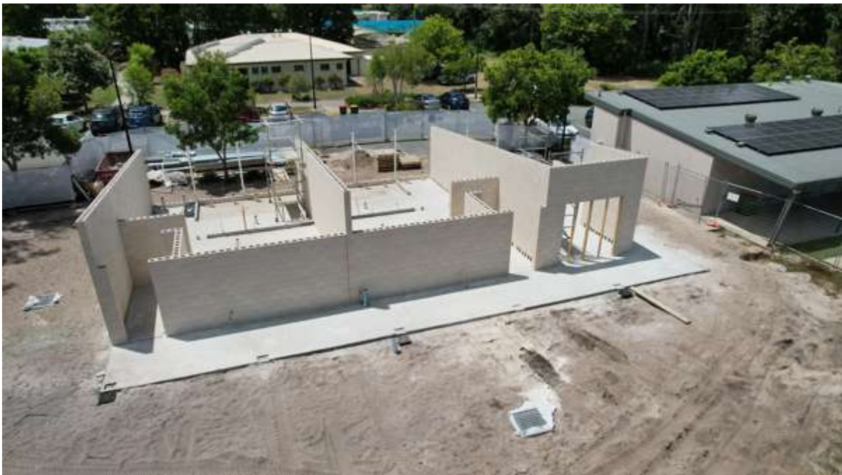
Blockwork completed
