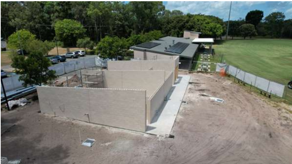
Blockwork completed
