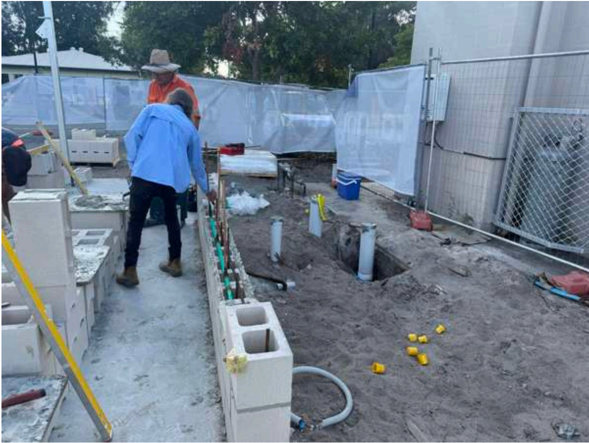
Installation of plumbing to water trough wall
