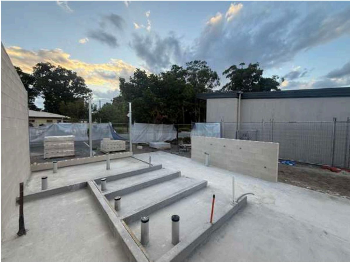
Blockwork nearing completion
