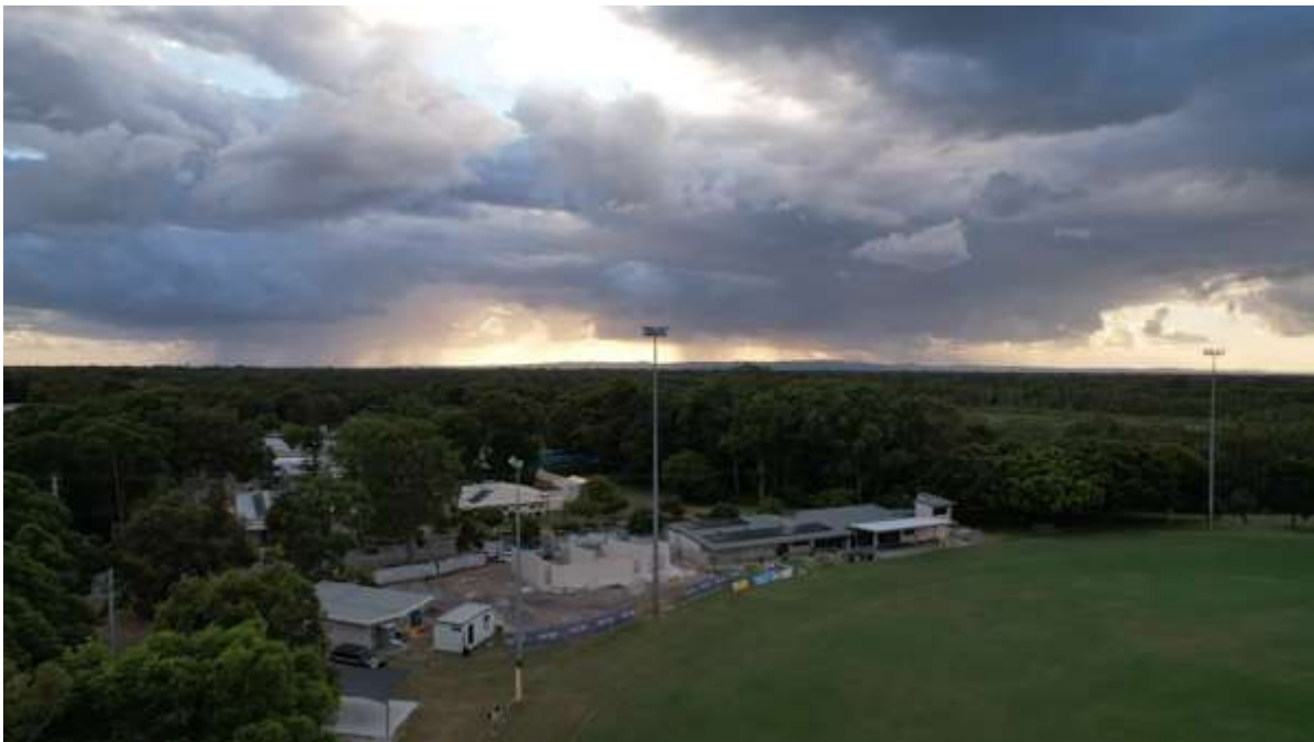
Overview of site
