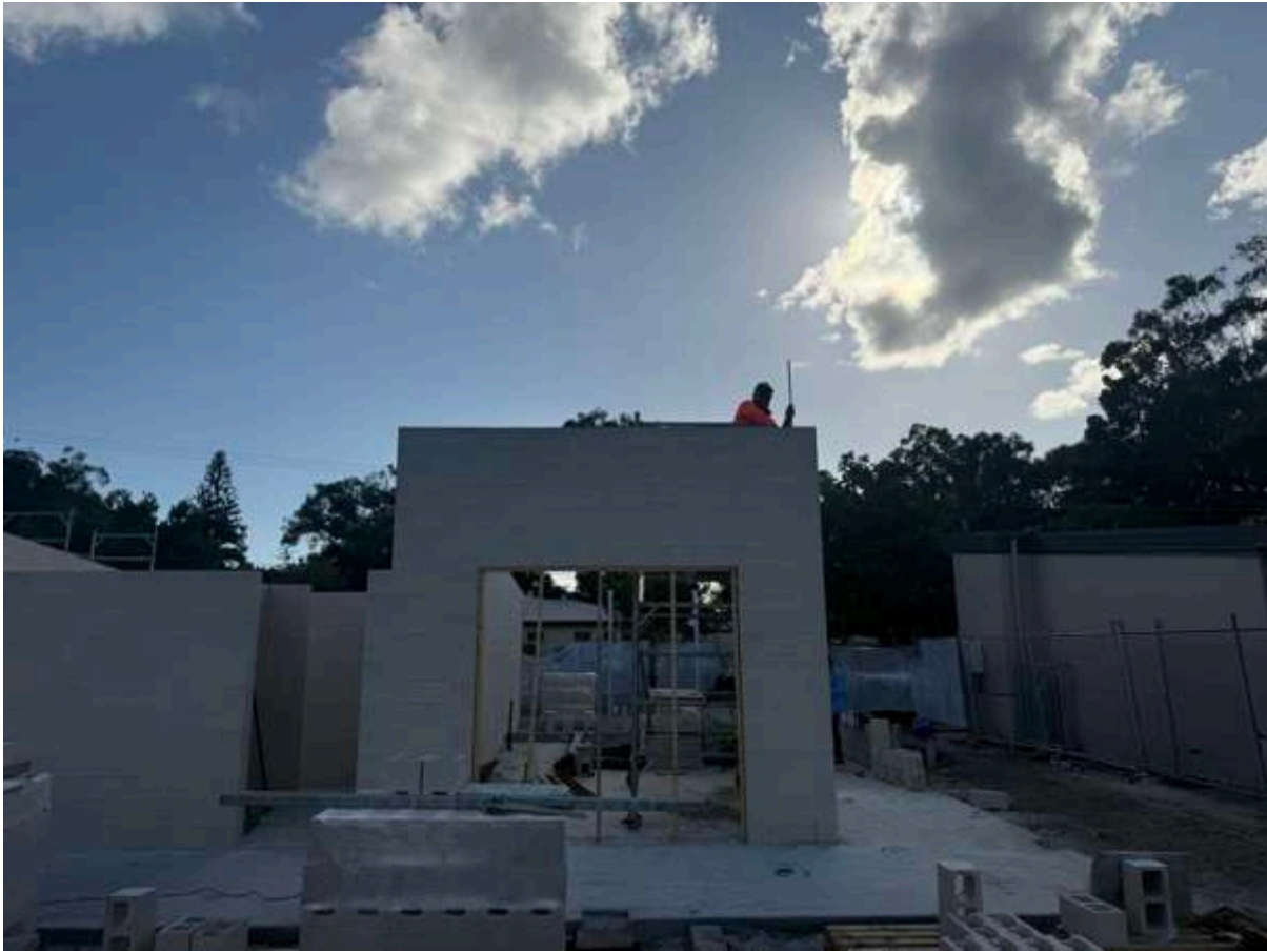
Installation of vertical steel reinforcement
