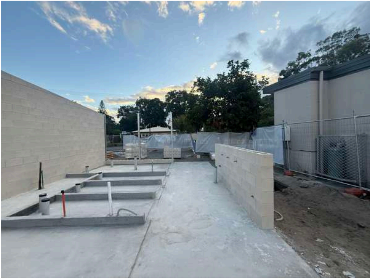
Blockwork nearing completion
