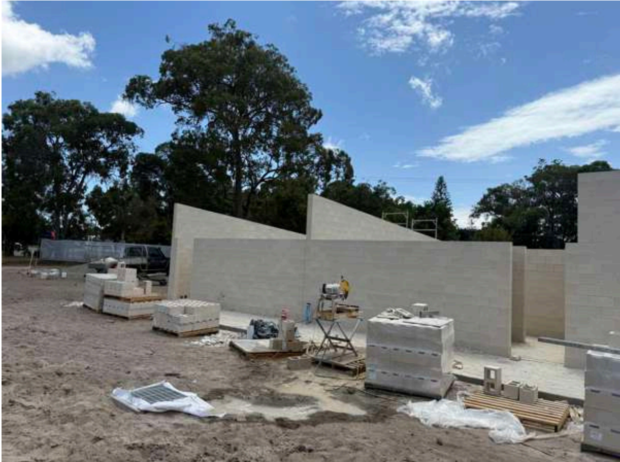
Construction of block walls
