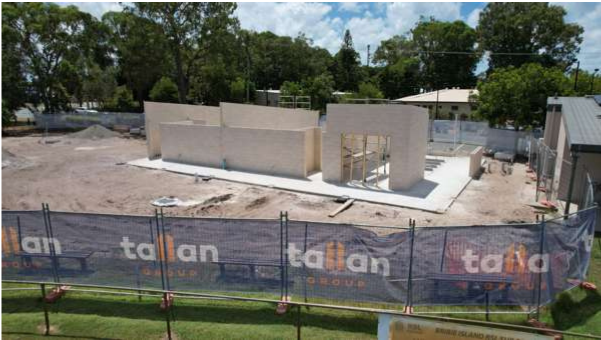
Blockwork completed
