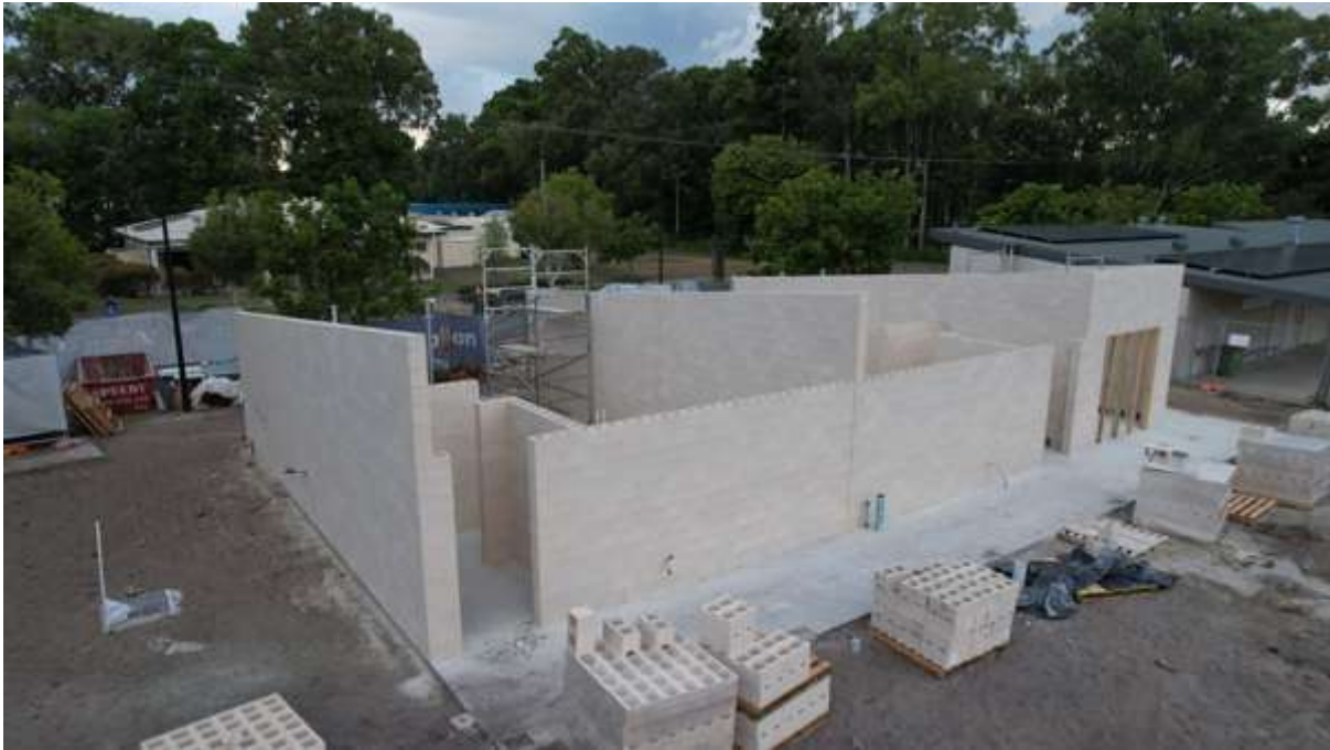
Blockwork nearing completion
