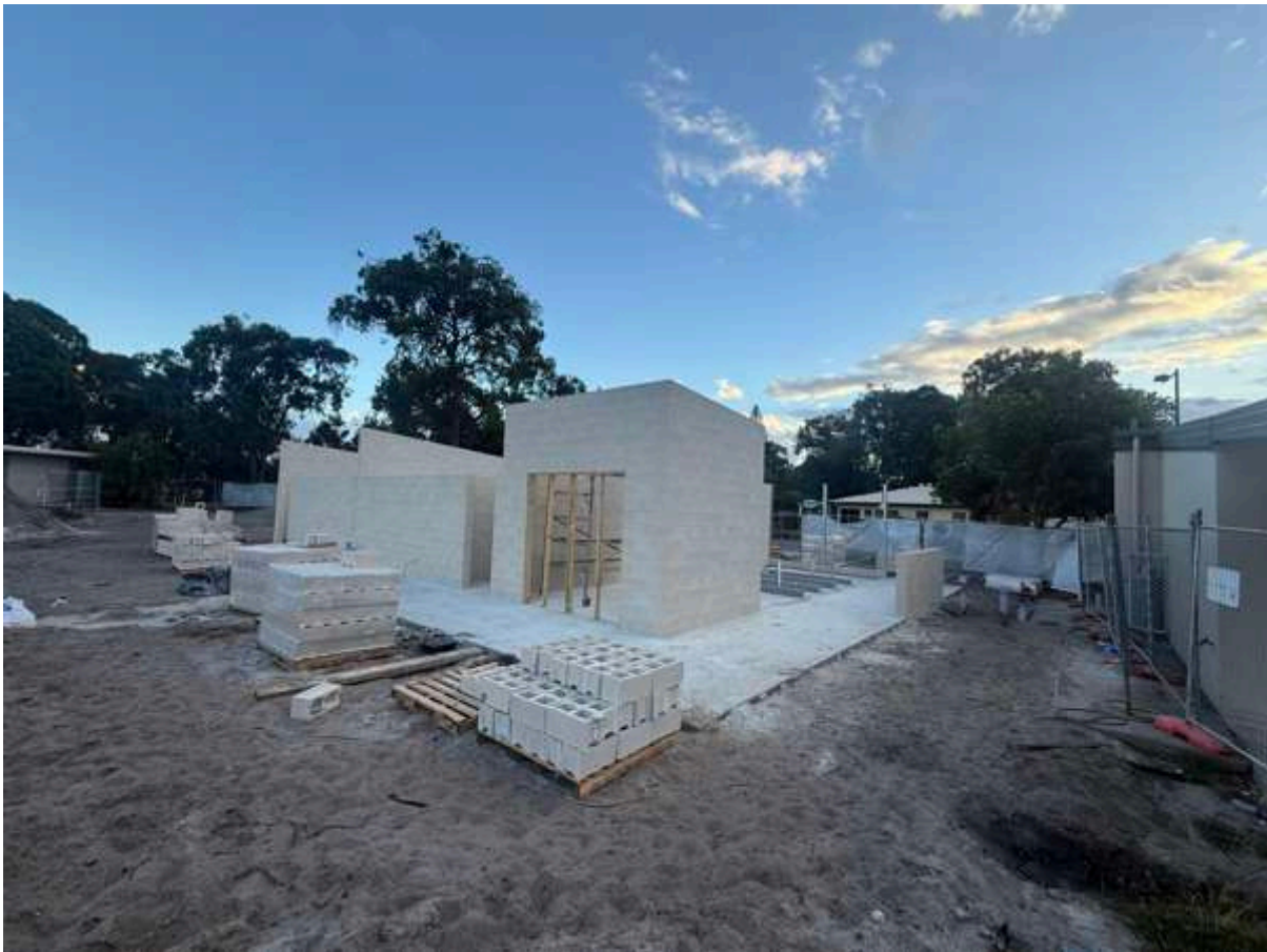
Blockwork nearing completion
